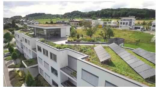
Green roof with solar panels
