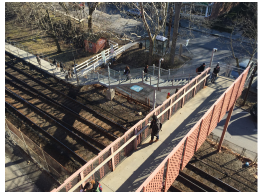
Pedestrian Bridge to Scarsdale Avenue
